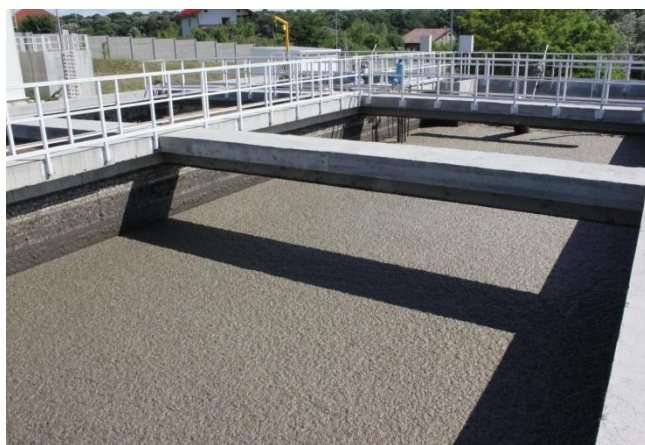
Treatment plant - Brănești
